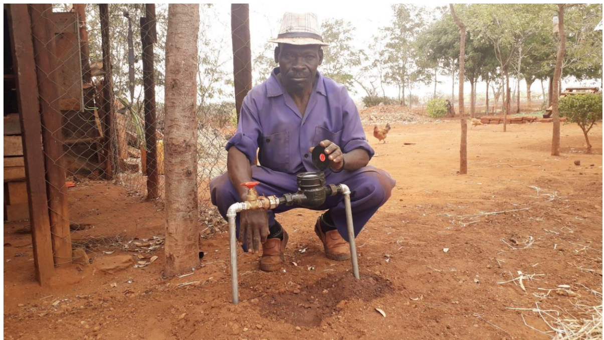
A view of a metered household connection
